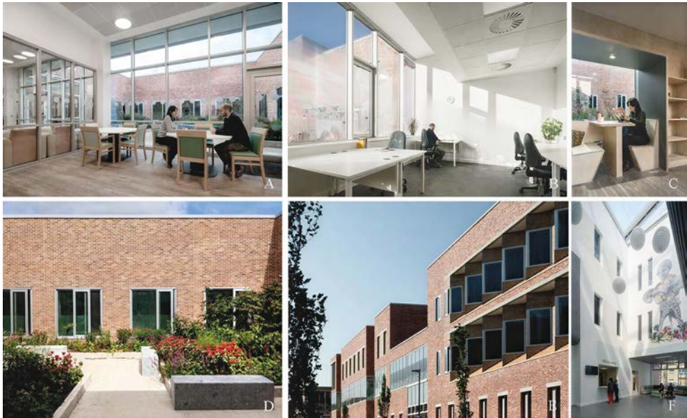
Fig. 9. Spaces and building elements providing access to daylight and fresh air: large glazed areas in halls and common areas (A, B, C); windows opening onto the courtyard (D); windows in each patient room (E); glass roof in communal areas (F) [C.F. Møller Architects, photo: Mark Hadden]
