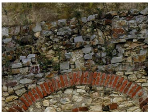
Photo 5 Southern enfilade, eastern part (Andrzej Firlej Palace). 2010.
