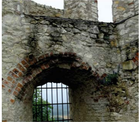
Photo 4 Wall connecting the gatehouse and the eastern tower. 2025.
