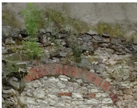
Photo 6 Southern enfilade, eastern part (Andrzej Firlej Palace). 2025.
