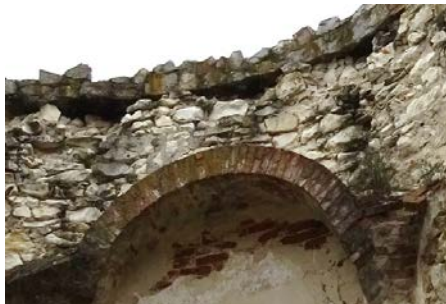
Photo 18 Quartzite capping of the chapel wall crest. 2025
