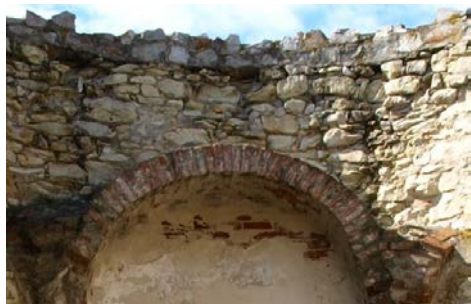
Photo 17 Quartzite capping of the chapel wall crest. 2010
