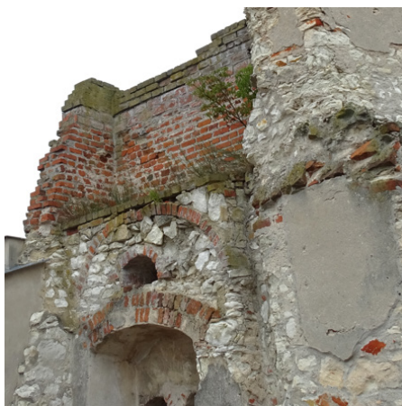
Photo 22 Wall connecting the Great Bastion and the Northern House. 2025.
