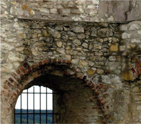
Photo 3 Wall connecting the gatehouse and the eastern tower. 2010.
