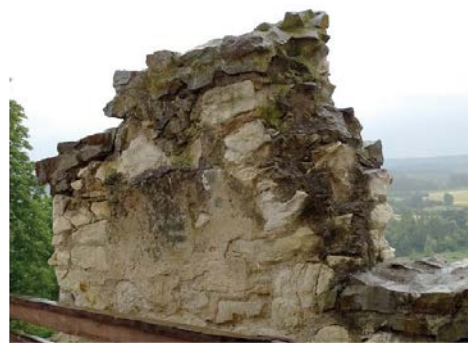
Photo 2 Wall of the gate neck. 2025.
