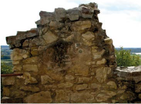
Photo 1 Wall of the gate neck. 2010.
