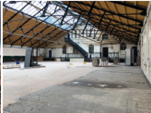
Fig. 6 Photograph of the Drill Hall interior.
