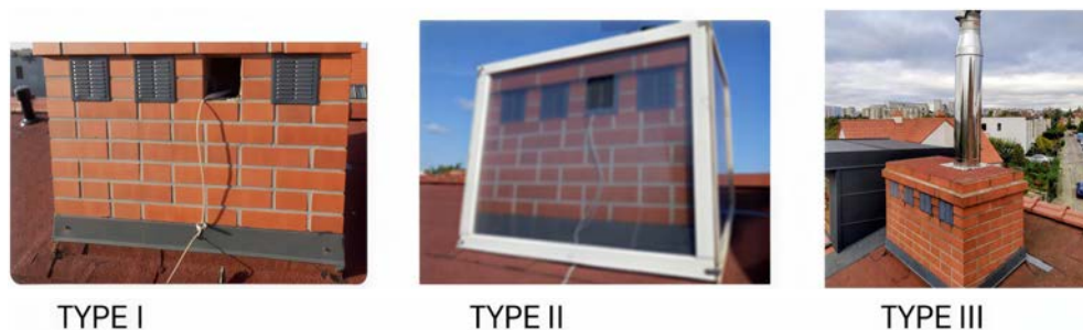
Fig. 3. Real type of the three chimney configurations (Type I – traditional, Type II – solar, Type III – rotary cap) [from the author's collection]
