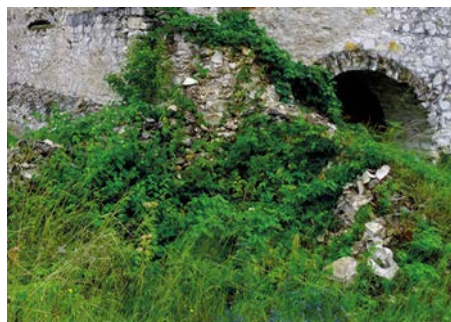
fig. 14. Remains of walls adjacent to the southern enfilade, western part (Tarło Palace), 2025
