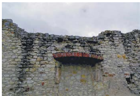
Fig. 26. Walls of the servants' quarters (northern outbuilding), 2025
