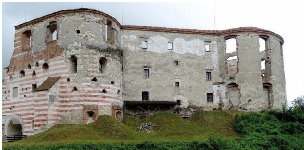
Fig. 5. Wall of the gate neck, 2010
