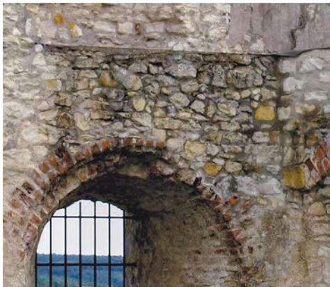
Fig. 9. Wall connecting the gatehouse and the eastern tower, 2010
