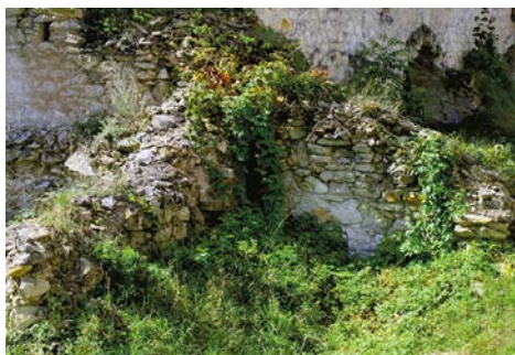
Fig. 13. Remains of walls adjacent to the southern enfilade, western part (Tarło Palace), 2010
