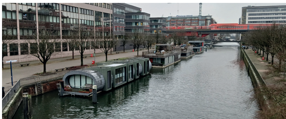
Fig. 5. Architectural proposals for the use of structures resistant to high flood waves implemented as part of IBA Hamburg: (from left at the top) (5a) amphibious buildings from the WaterHouses programme, (5b) the IBA Dock office building, and (5c) the die Mügge community centre [own source]
