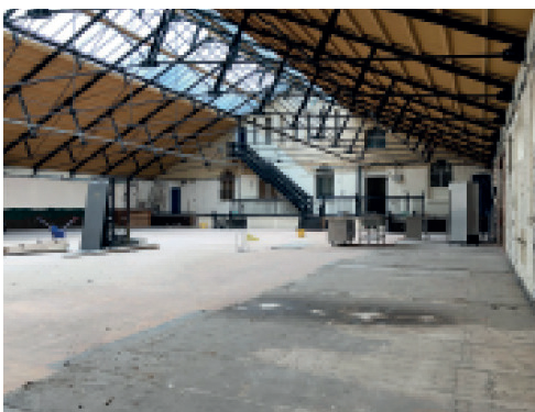
Fig. 6. Photograph of the Drill Hall interior [photo authors]
