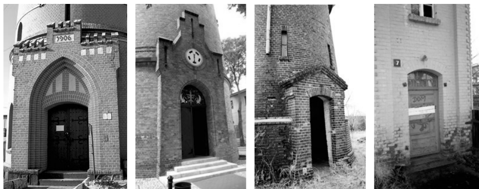
Fig. 3. Entrance area of the water tower in (from left): Nowe, Toruń, Chełmża, Lniano [photo: Piotr Brzeziński]
