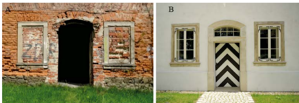
Fig. 32. Reconstruction of windows and doors and restoration of façade: 2018 (A); 2024 (B) [Archives of the Department of Conservation of Monuments]
