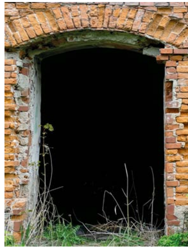
Fig. 15. Ceramic brick lintel
