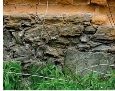
Fig. 14. The plinth of broken stone
