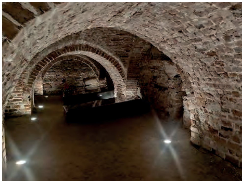
Fig. 6. Underground of the Cathedral in Drohiczyn [Chelm.naszemiasto.pl 2024]
