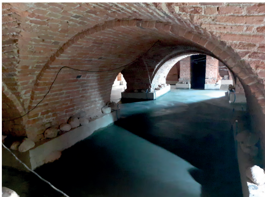
Fig. 21. Crypts after completing the reinforced concrete slab, photo by A. Kieliszek
