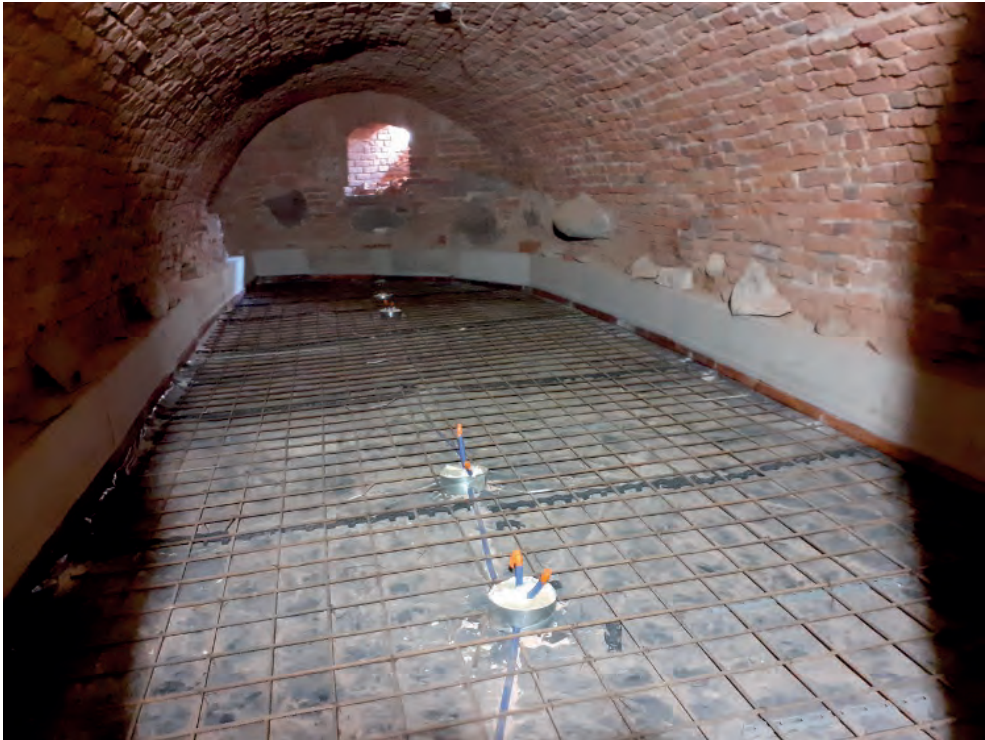
Fig. 20. Crypts after reinforcing the slab, photo by A. Kieliszek
