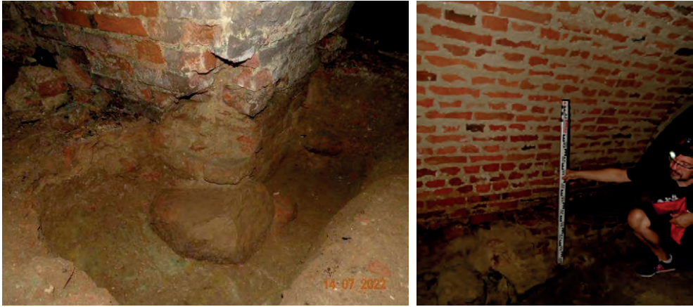
Fig. 15. Technical condition of the foundations (A) and crypt height before adaptation (B), 2022, photo by B. Szostak
