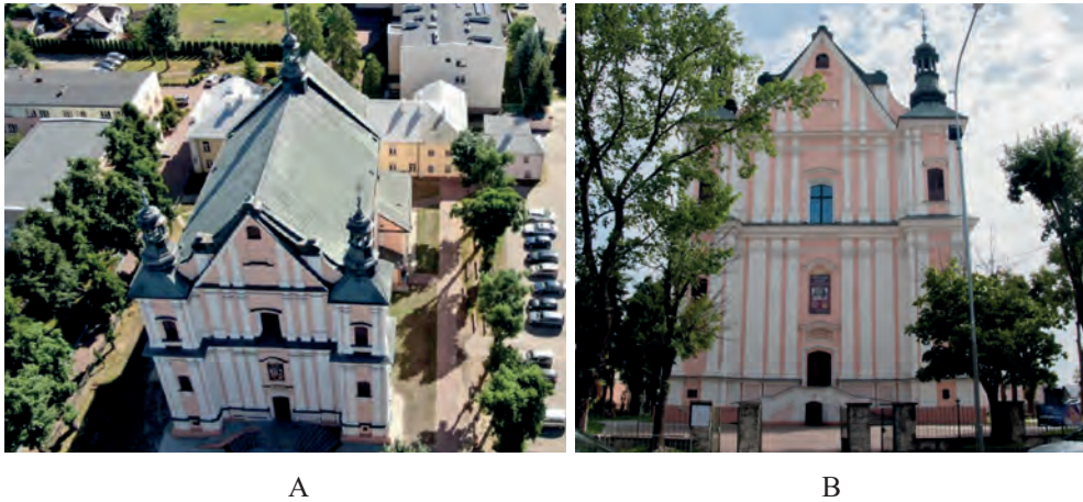
Fig. 5. Church structure from the west (A) and the current view of the front façade (B), 2022, photo by B. Szostak
