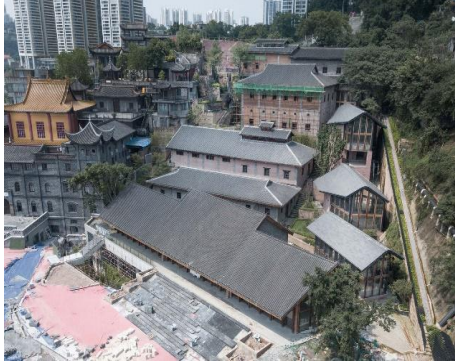
Fig. 5. Bird view of the site (from the authors)
