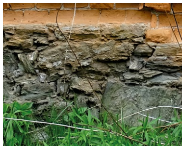
Fig. 14. The plinth of broken stone
