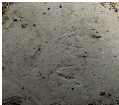
Fig. 27. Floor, casemate no. 1
