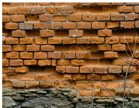
Fig. 13. Exterior wall in ground level strip
