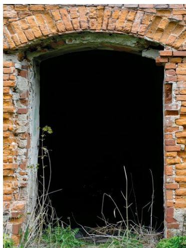
Fig. 15. Ceramic brick lintel
