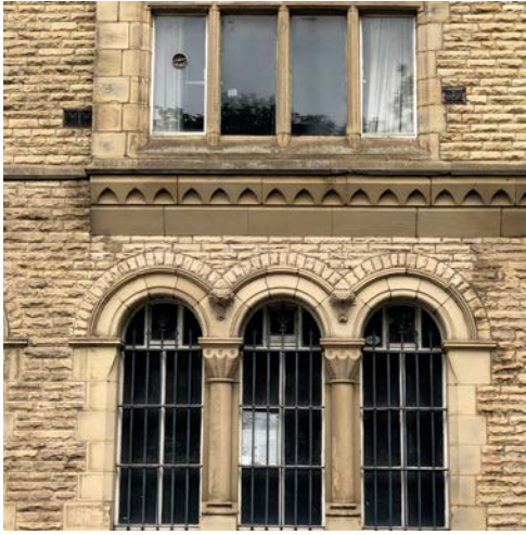
Fig. 13 Photograph of details of the existing facade. [Source: photo authors]
