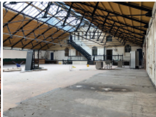
Fig. 6. Photograph of the Drill Hall interior [photo authors]
