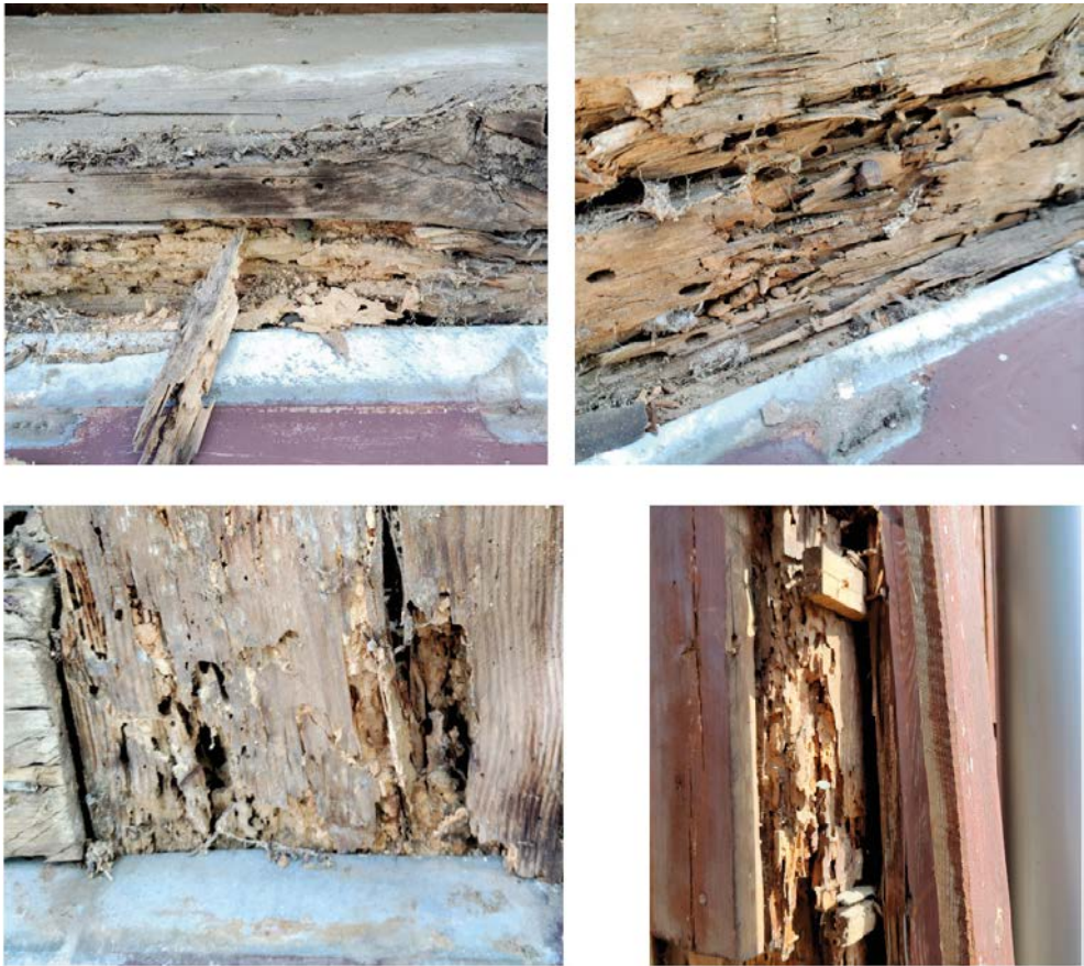
Fig. 2. Photographs illustrating damage caused by infestation by the house longhorn beetle and the common furniture beetle – [photo by M. Trochonowicz]
