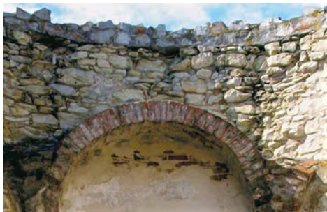
Fig. 23. Quartzite capping of the chapel wall crest, 2010
