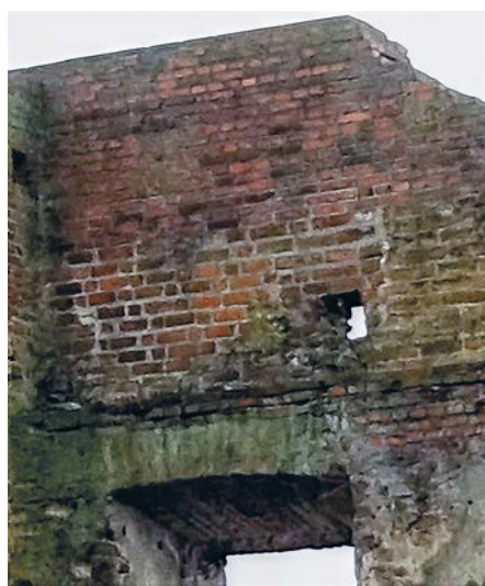
Fig. 16. Southern residential tower (southern risalit), 2025
