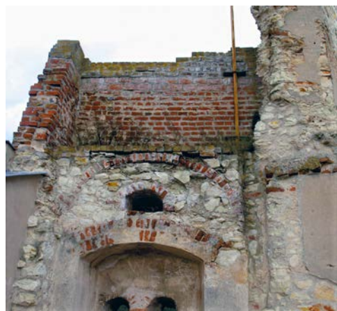
Fig. 27. Wall connecting the Great Bastion and the Northern House, 2010
