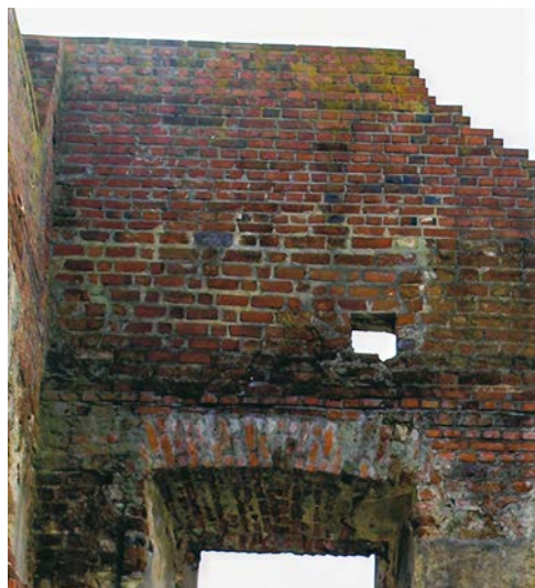
Fig. 15. Southern residential tower (southern risalit), 2010
