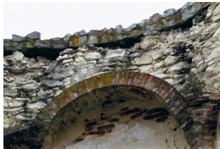
Fig. 24. Quartzite capping of the chapel wall crest, 2025
