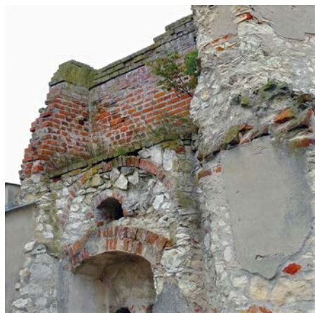
Fig. 28. Wall connecting the Great Bastion and the Northern House, 2025
