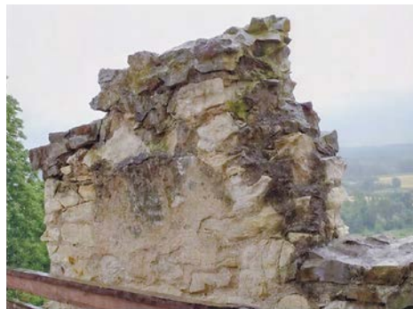
Fig. 8. Wall of the gate neck, 2025
