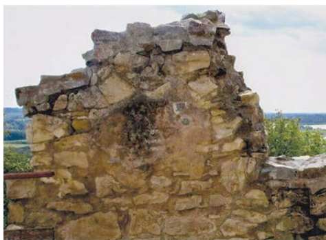
Fig. 7. Wall of the gate neck, 2010
