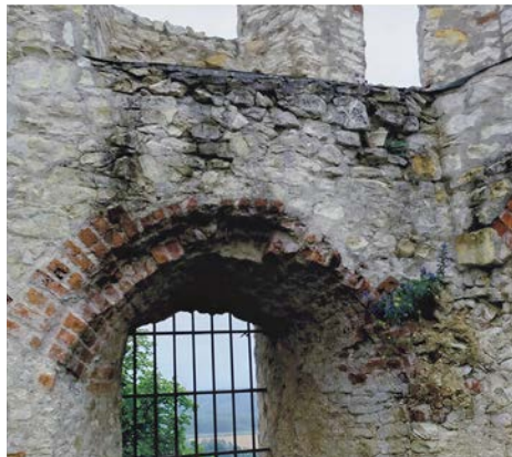
Fig. 10. Wall connecting the gatehouse and the eastern tower, 2025
