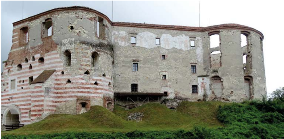
Photo 1 Wall of the gate neck. 2010.
