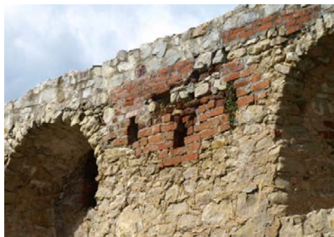
Photo 11 Northern defensive wall. 2010.
