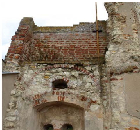
Photo 21 Wall connecting the Great Bastion and the Northern House. 2010.
