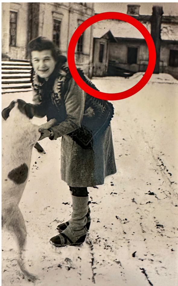
Fig. 3. The only historical photo found to show a fragment of the no-longer-existing original orangery that connected the manor house and the outbuilding (highlighted in red) [current owners' archive, photo found during the manor house survey]
